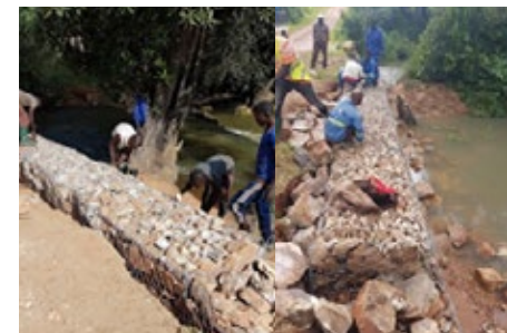
Mwaleshi bridge retaining wall construction in dry season
