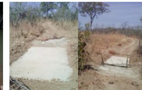
Bed-level drifts to enable year-round access throughout the Rhino Conservation Area
