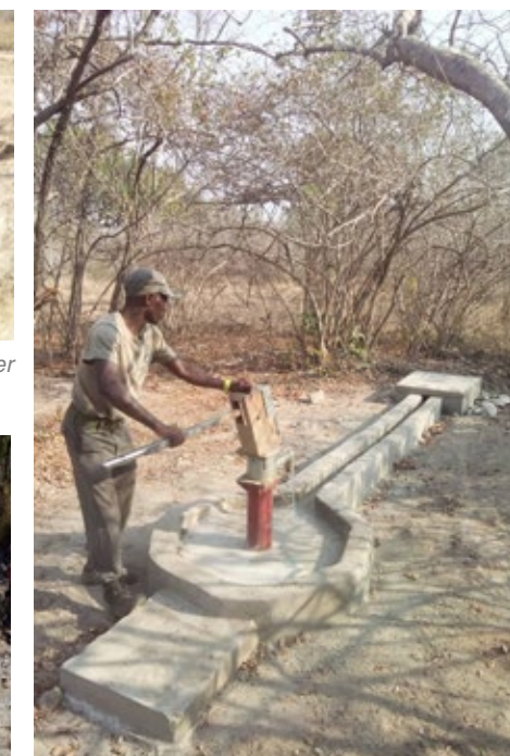
Boreholes constructed at the new scout picket locations
