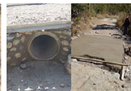
Access to Mwaleshi Picket improved with construction of a culvert drift
