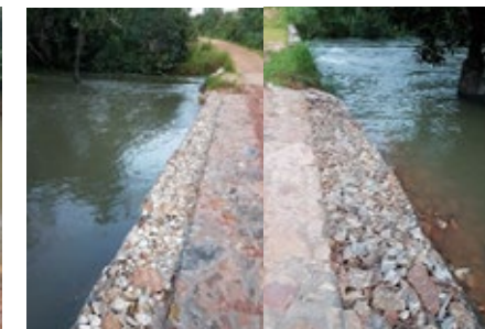
Completed works and Mwaleshi River in flood
